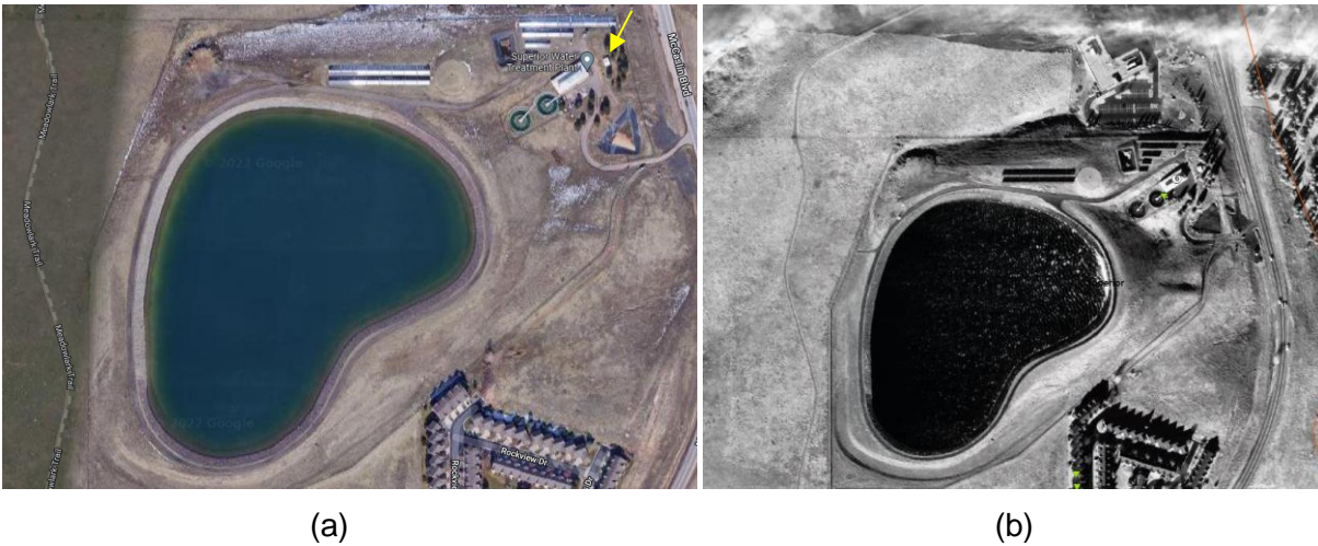
Figure 7-4. Superior WTP overhead (a) google earth image showing location of destroyed backup generator and (b) at 2 PM 12/30 with fire to the north (39°56'33.8" N, 105°09'50.2" W)
