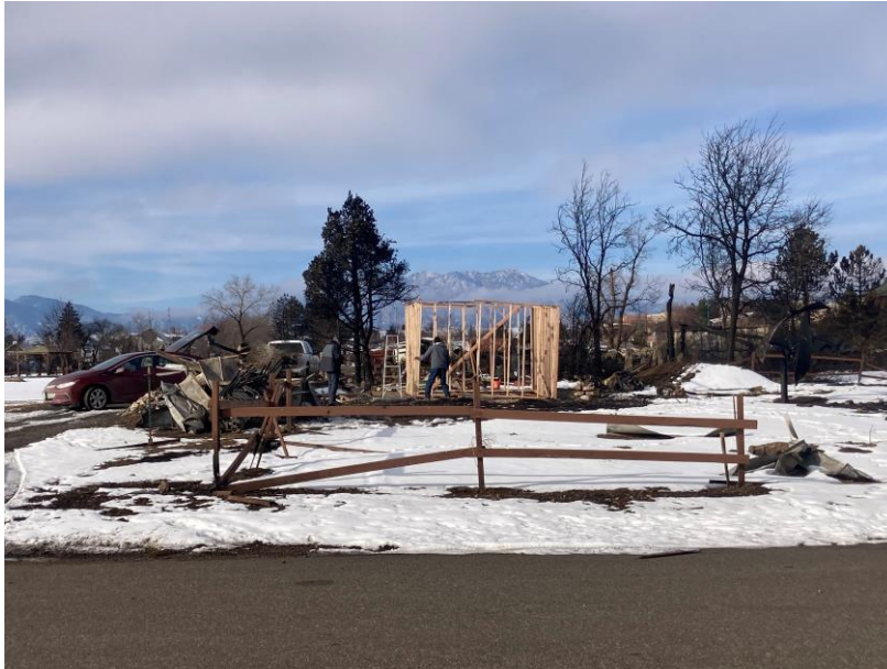
Figure 8-25. Initial signs of rebuilding, Original Town Superior, 9 January 2022 (39.95383, -105.16684)
