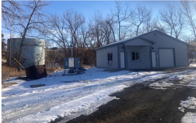
Figure 7–7. Sans Souci Mobile home park water station (39°57'24.8" N, 105°13'56.3" W)
