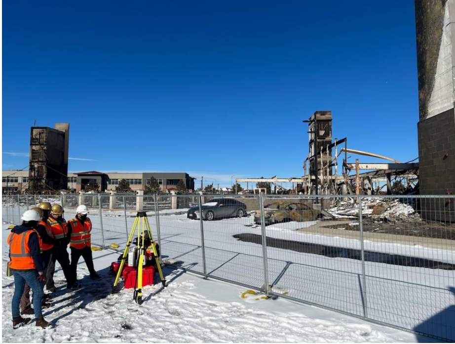
Figure 8-27. RAPID staff teaching students during LiDAR scans of Element Hotel (39°57'19.1" N, 105°09'48.7" W)
