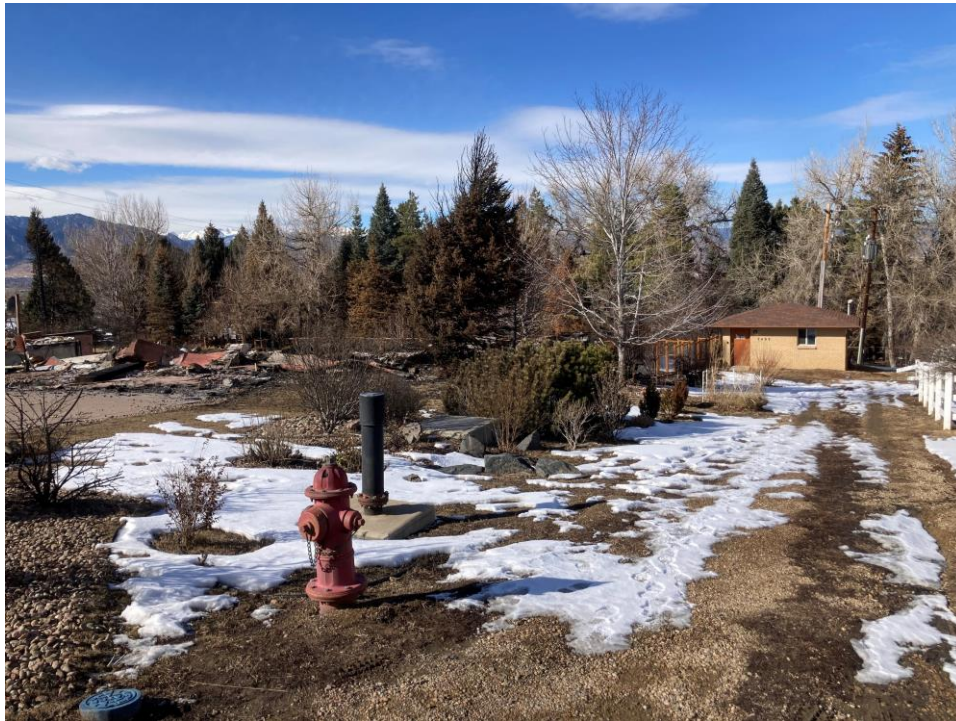
Figure 7–6. EBCWD Pump house with buried storage water tank in the foreground, adjacent to destroyed home (39°58'33.2" N, 105°10'40.8" W))
